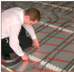
Below floor slab.
